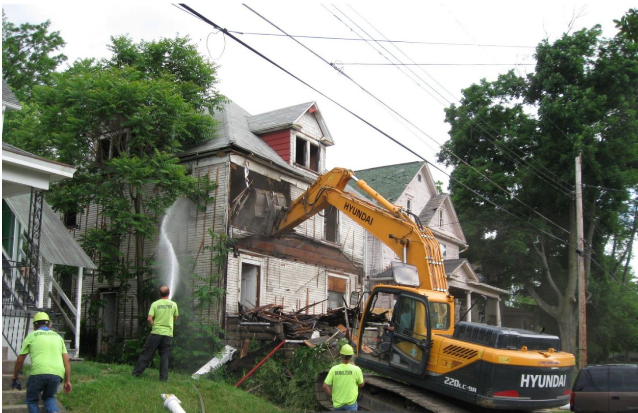
"In-Process" Demolition Photo, Alliance, OH
