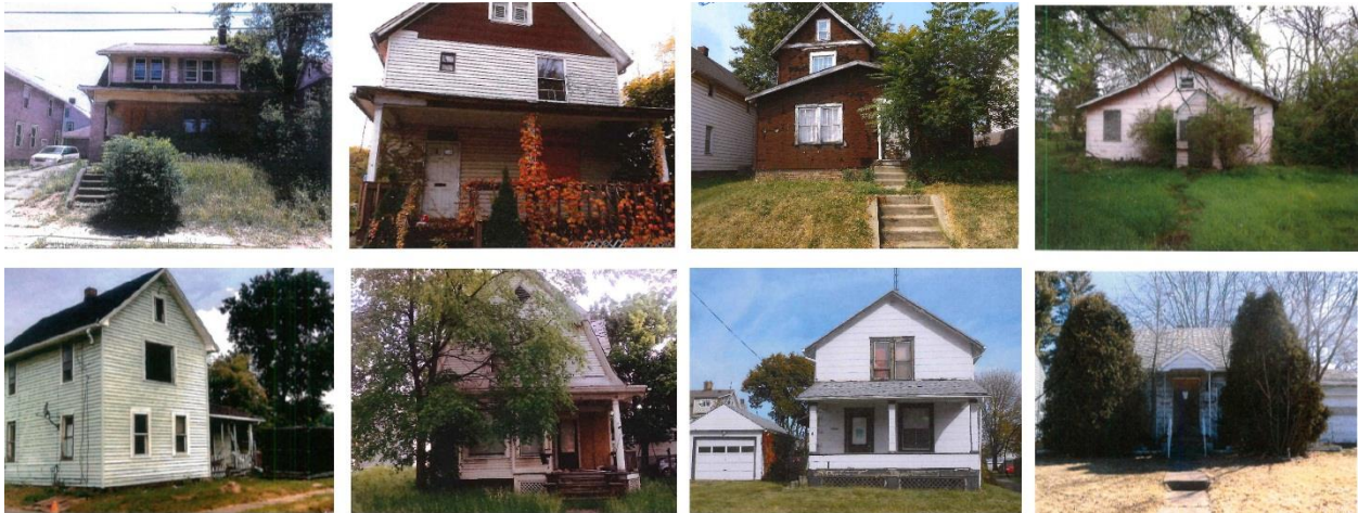
"Before" photos of SCLRC owned properties located in Canton, OH
